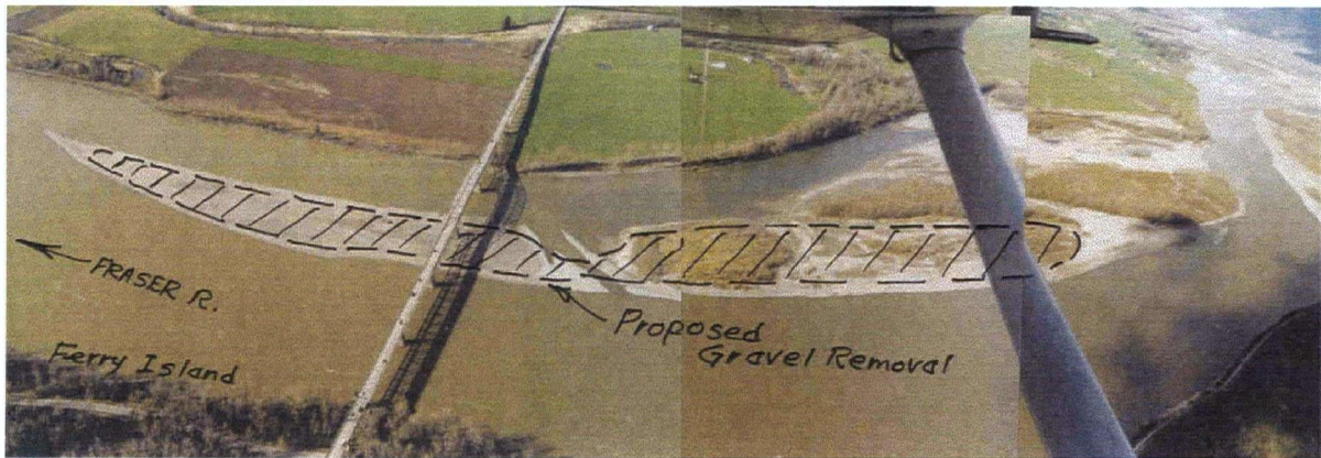
Figure 7.18: Proposed gravel removal area to reduce downstream bank erosion (after Northwest Hydraulic Consultants Ltd., 1999)
