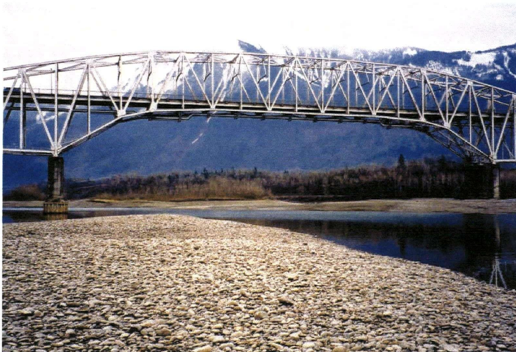
Figure 6.3: Fraser R.: Agassiz-Rosedale Bridge looking upstream at Q = 650 \text{ m}^3/\text{s}
