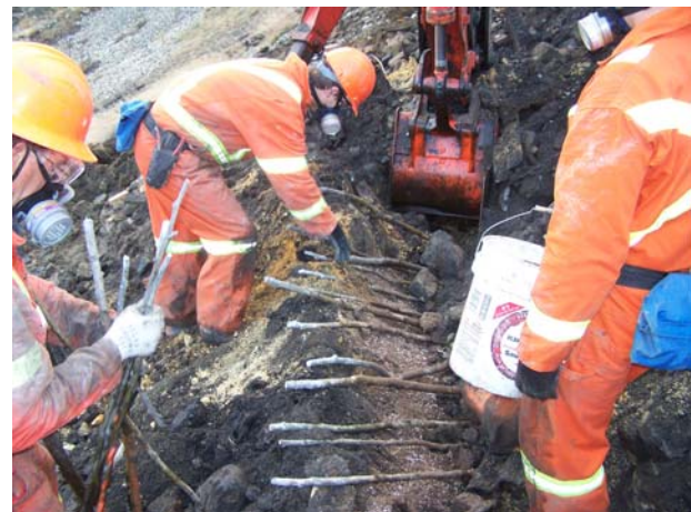
1-8 Placement of cuttings in trench. Unit 3 Nov. 2006.
