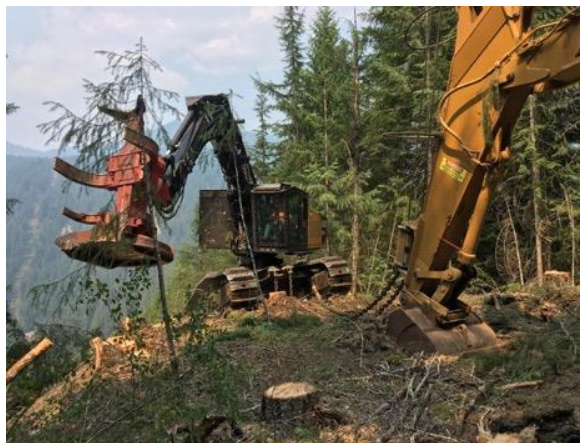
Figure 2. Cat 552 Feller-Buncher tethered to an excavator with a shovel embedded in the ground operating in steep slope terrain (Siegmond Excavation, 2018).
