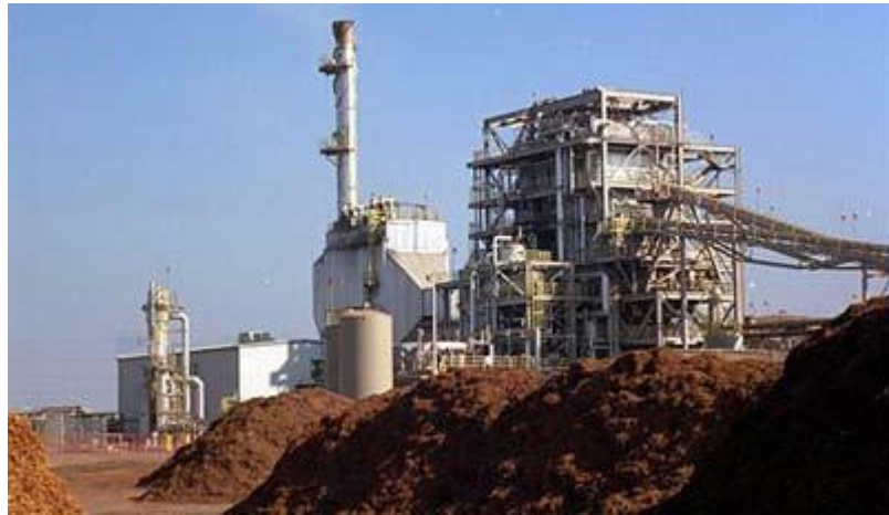
FIGURE 1: A BIOMASS POWER PLANT THAT UTILIZES WOOD WASTE
