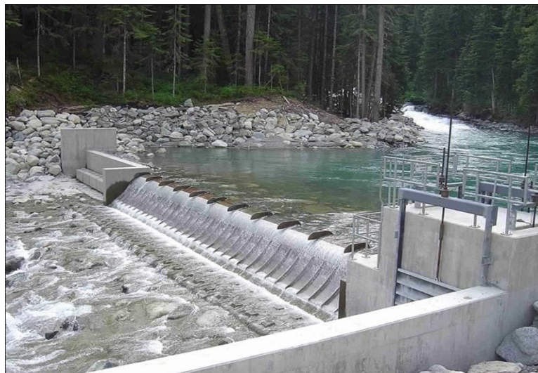
FIGURE 4: INTAKE STRUCTURE FOR A RUN-OF-RIVER PROJECT
