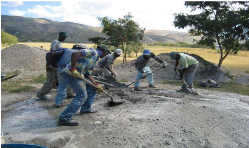
Figure 4: Illustrating ground mixing of cement mixing in Haiti
