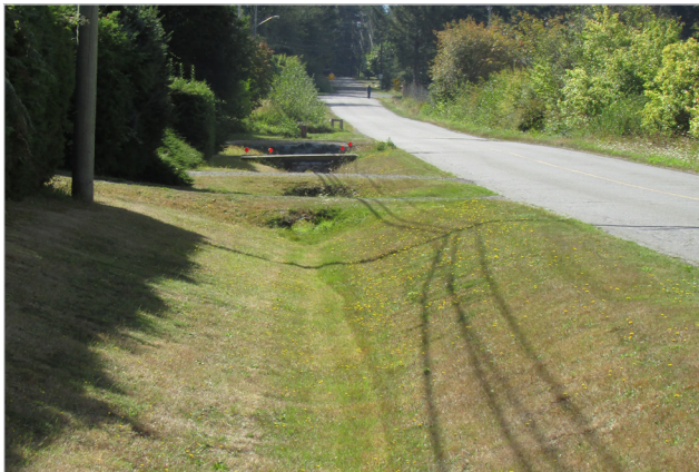
Figure 7. Roadside ditch part of the electoral area's rainwater conveyance system. Photo credit: Jenna Cook
