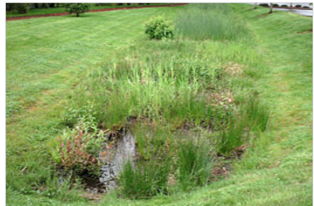
Figure 15. Neighbourhood scale detention pond. Photo credit: Stormwater Partners of Southwest Washington. 42
