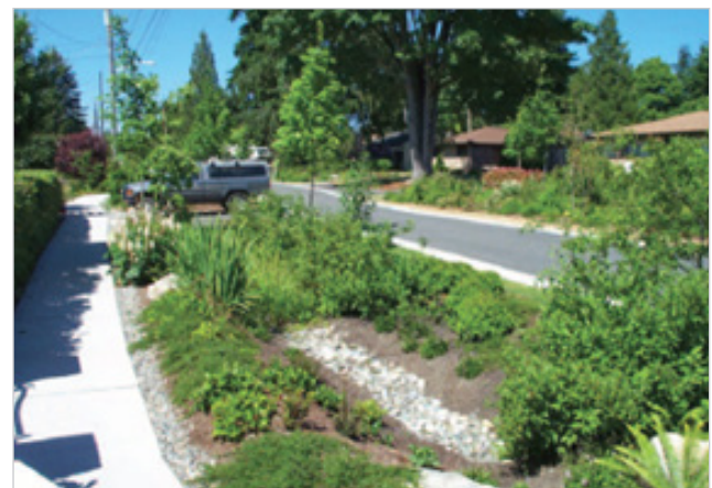
Figure 16. Neighbourhood scale bioswale adjacent to a road. Photo credit: City of Seattle. 35
