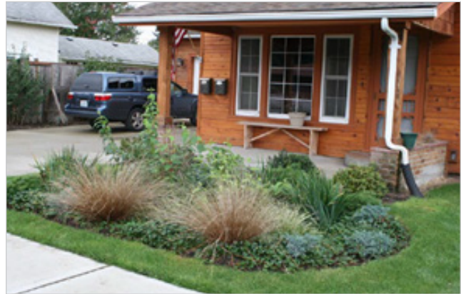
Figure 14. Rain garden on a single-family lot. Photo credit: Rain Dog Designs. 41
