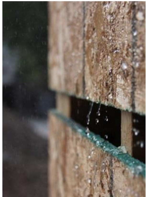
Figure 2.3. A single-family home under construction in West Point Grey, Vancouver, Canada (left). The mud and water in the foreground suggests that the building was exposed to rain water. A close up (right) of OSB wall sheathing that was left unprotected in a rain shower, while the building was under construction
