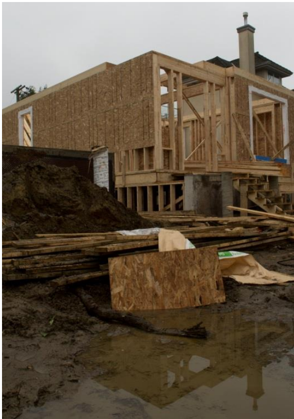
Figure 2.3. A single-family home under construction in West Point Grey, Vancouver, Canada (left). The mud and water in the foreground suggests that the building was exposed to rain water. A close up (right) of OSB wall sheathing that was left unprotected in a rain shower, while the building was under construction
