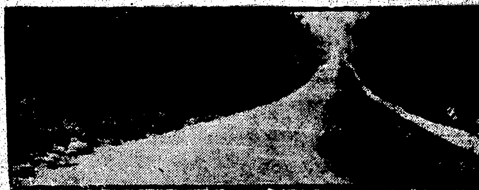
Bitulithic Paving on Marine Drive
