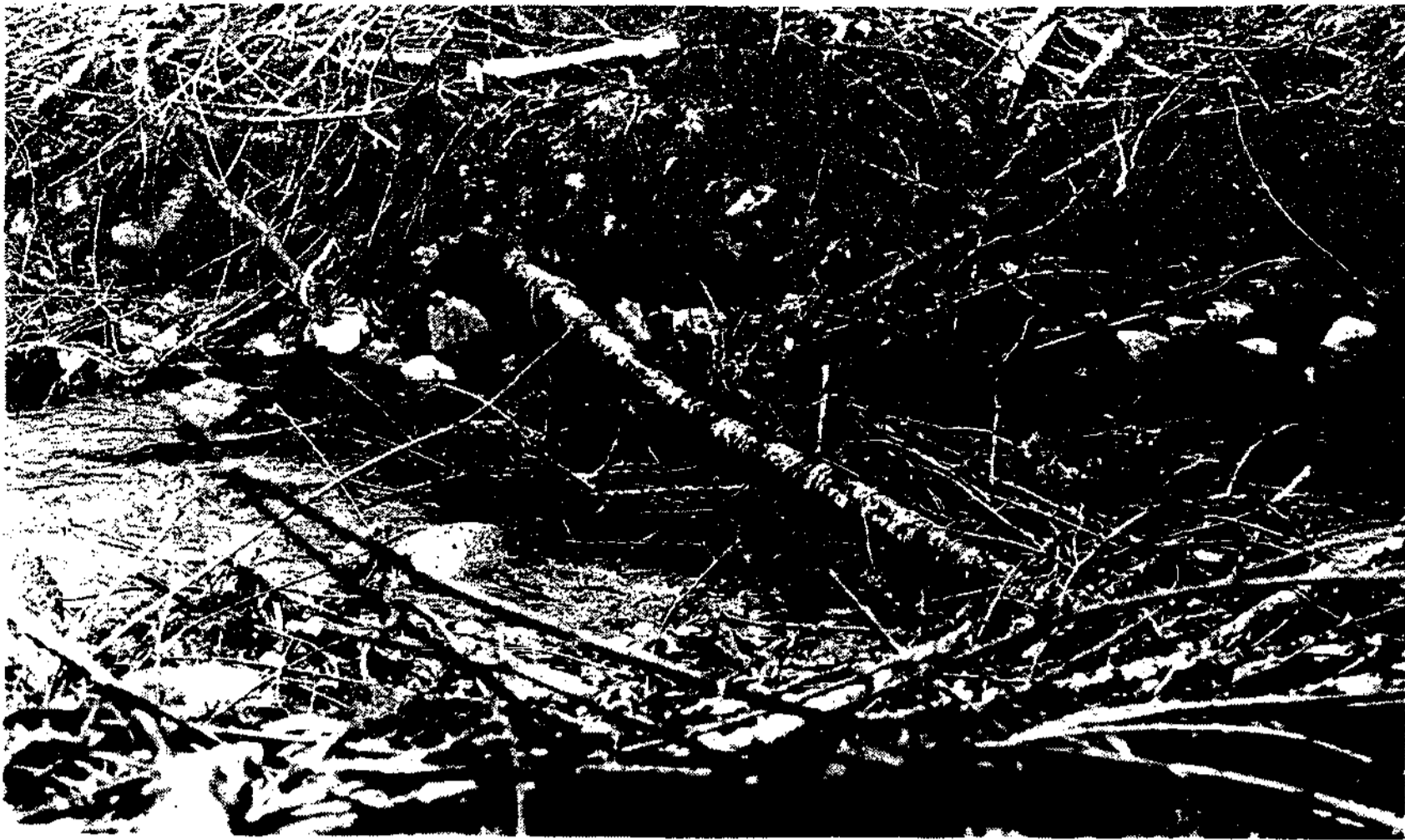
The picture shows the cause of Fisheries Officer Ray Kraft's concern about Twin Creek, blocked by careless work by a Department of Highways crew clearing a road
