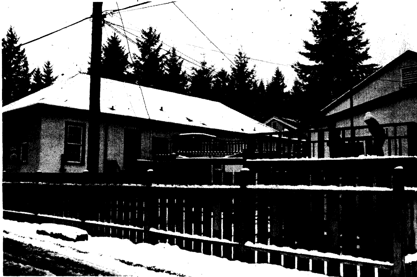
UBC's child care facilities at Acadia Camp have been threatened with closure because the 40-year-old army huts are a fire hazard. Renovating them or replacing them would cost about $1 million, but government policy is "no money for child care facilities."
