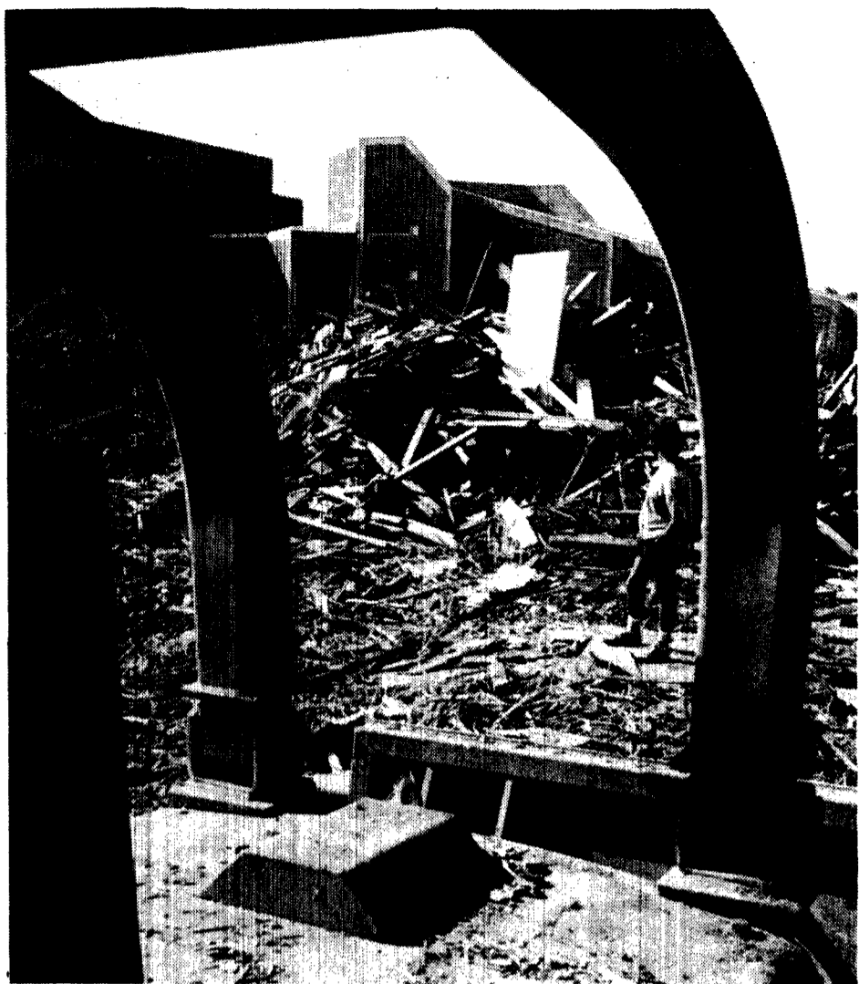
Surveying the ruins of the East Mall Classroom Annex, known as EMAX to its occupants, is a Faculty of Law student who said he once attended lectures in the building. By the time you read this, a new 52-car parking lot will be nearing completion on the site.
