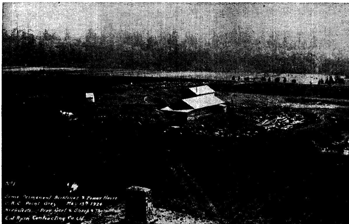
TWO-YEAR-OLD STONE CAIRN commemorates the G reat Trek, while several acres of cleared land and construction shacks hold the promise of the future for the 1451 students then attending classes at the young University of British Columbia. Picture was taken from the top of the Chemistry Building in 1924. For later pictures from the same point see pages three and four.
