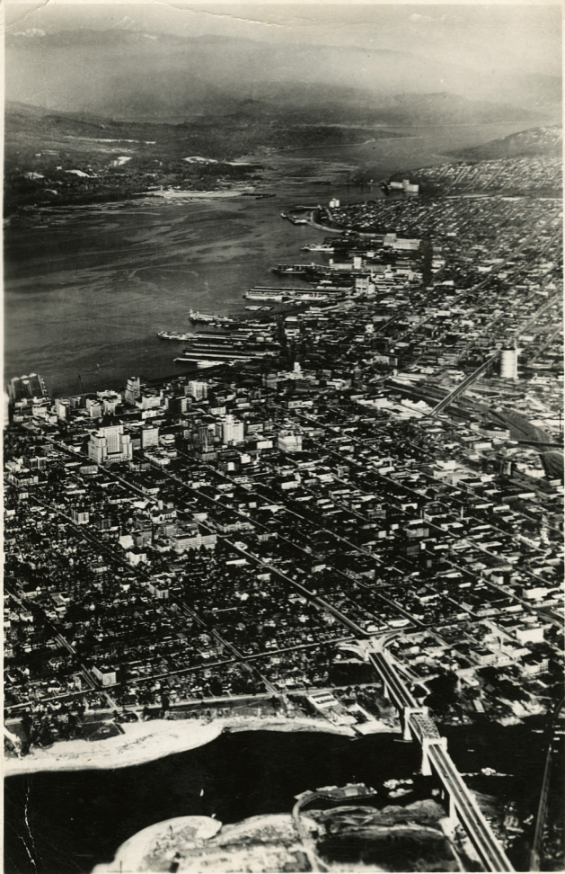
VANCOUVER AND BURRARD STREET BRIDGE
