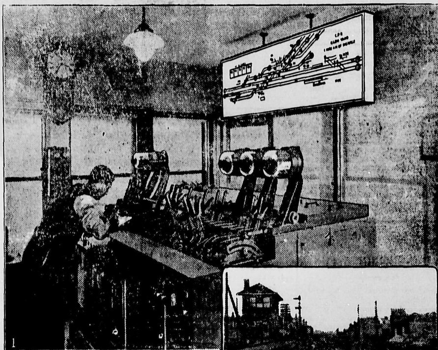
Above.—Interior of the Canadian Pacific Westmount interlocking tower, showing the control levers and the illuminated plan, the light bulbs appearing as black spots.
