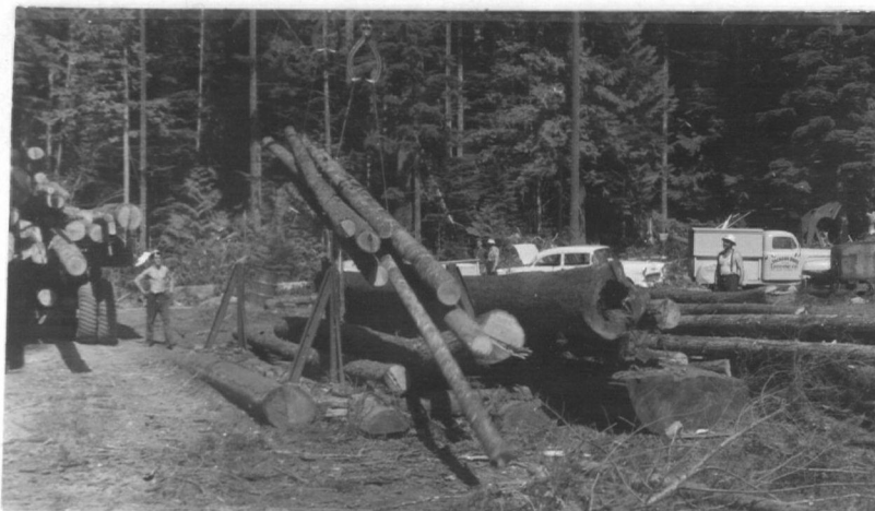
Fig. 19. Loading logs into a bundling bin. Sechelt tree farm.
