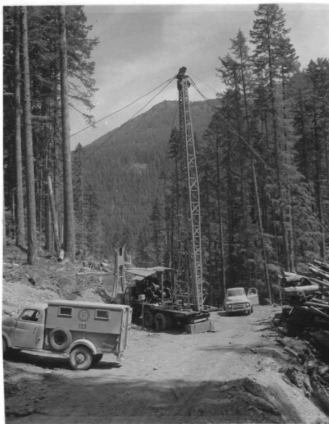
Fig. 26. Truck mounted mobile spar used for salvage and pre-logging.
