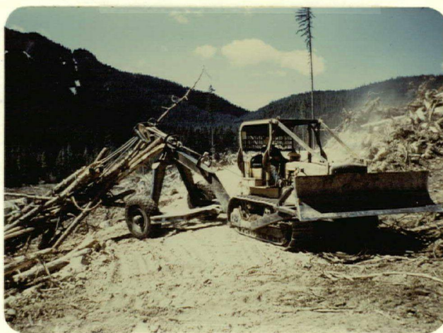
Fig. 14. D.6 tractor and arch logging salvage.
