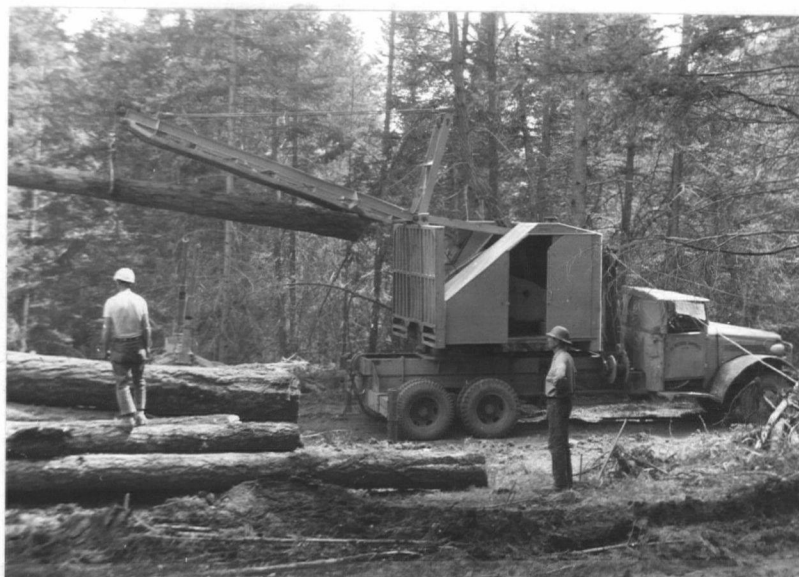
Fig. 54. Truck mounted Bohemian Boom Loading Crane. Note supporting guys.
