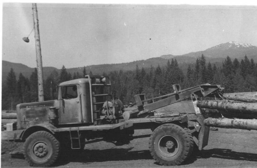
Fig. 44. Pacific 4x4 truck-arch. British Columbia interior.
