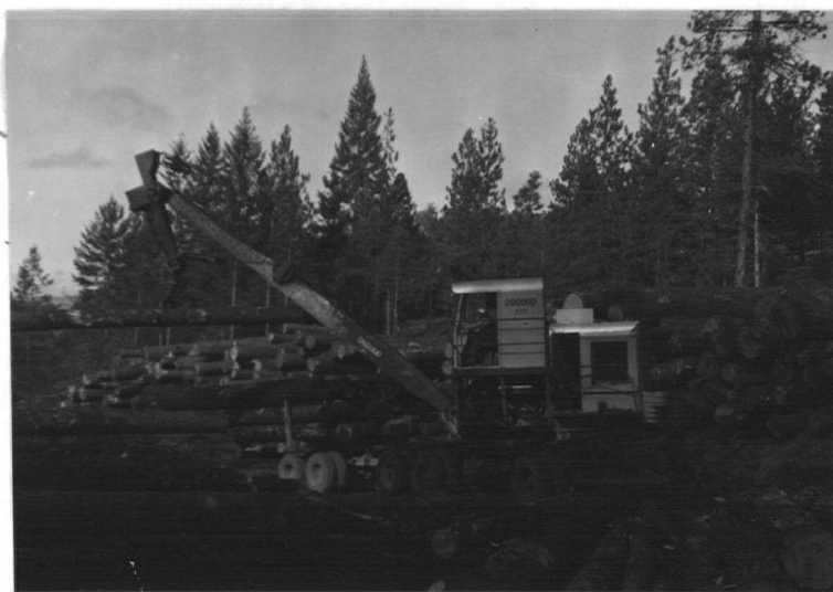
Fig. 18. Osgood loader with cab extended for better visibility.
