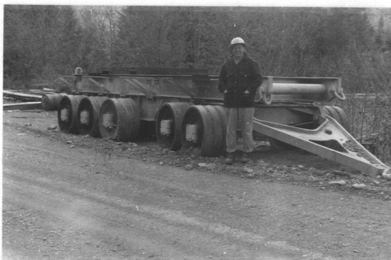
Fig. 49. Yarder chassis on discarded railway wheels with cut flanges.
