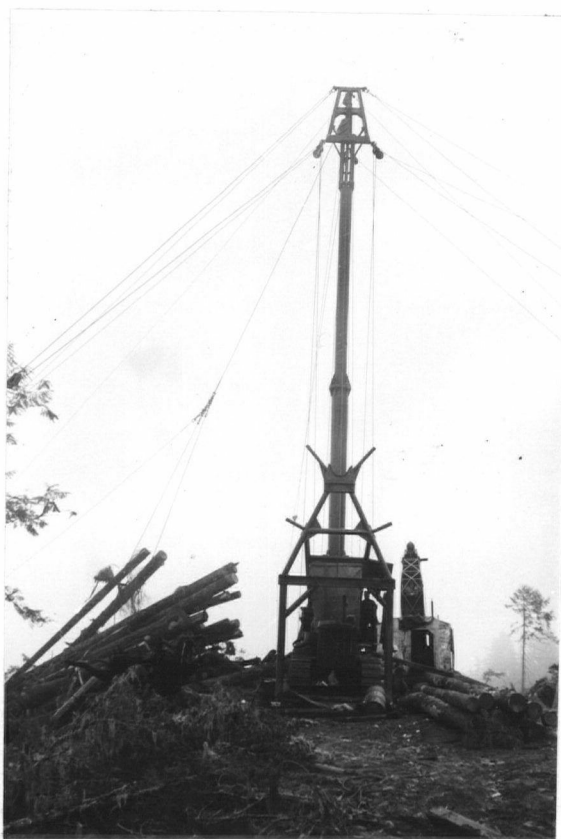
Fig. 37. Burrard 70' portable sled-mounted steel tower.
