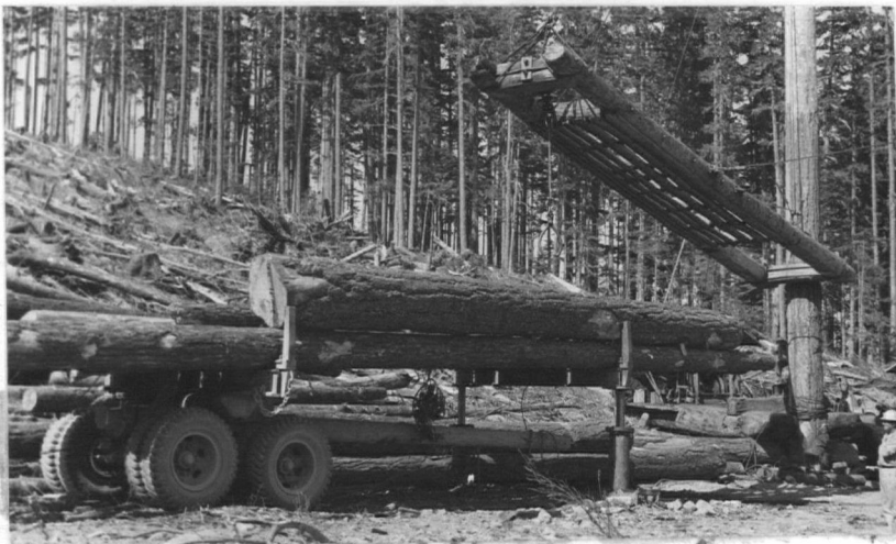
Fig. 47. Hydraulically operated pre-load device. Power from loader on right.
