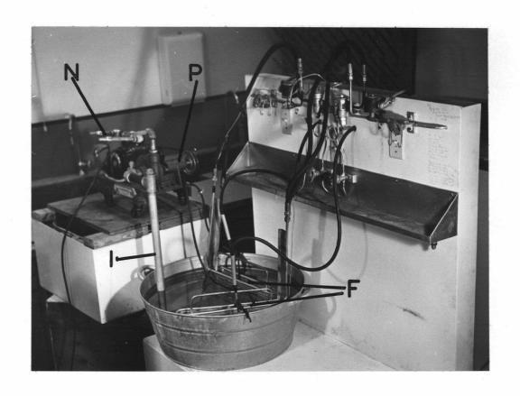
Figure 2. Apparatus used to pump a constant volume of water of required temperature through experimental troughs. P, 1/4 horsepower G.E. centrifugal pump; I, intake pipe; N, nozzles; F, twin coil Parmetic freezing unit.
