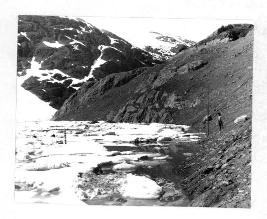
Figure 13: Staff gauges to record the rate of rise of the water surface of Summit Lake.
