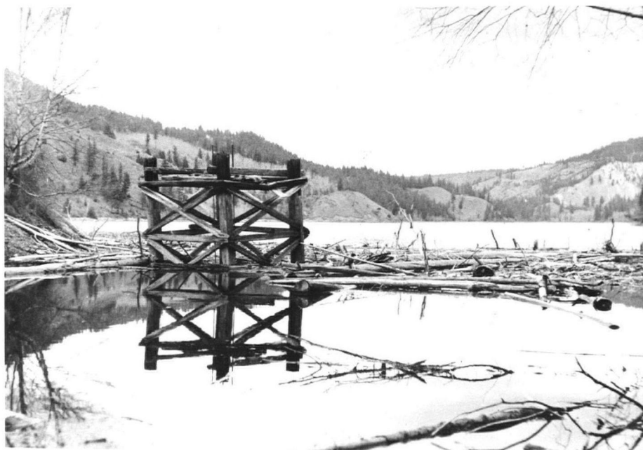
Photo 21. View of Snohoosh Lake from the dam. Construction in foreground shows the flood control gate in disrepair.
