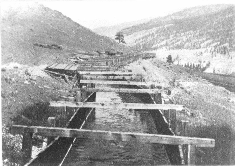
Photo 22. Main flume indicating flimsy construction
