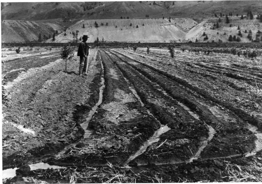
Photo 28. An example of the four-furrow system used to irrigate the orchards at Walhachin.
