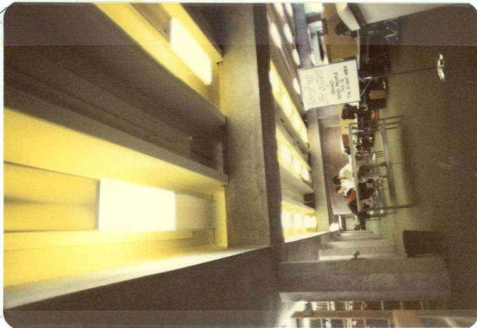
Figure 23 Pre-cast concrete ceiling
