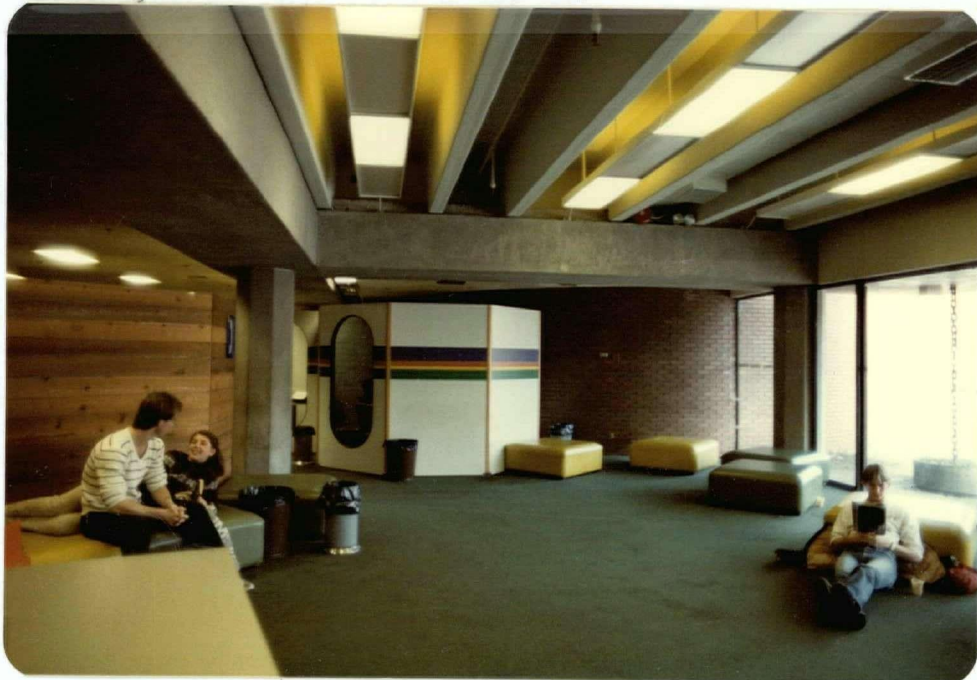
Figure 23 Pre-cast concrete ceiling
