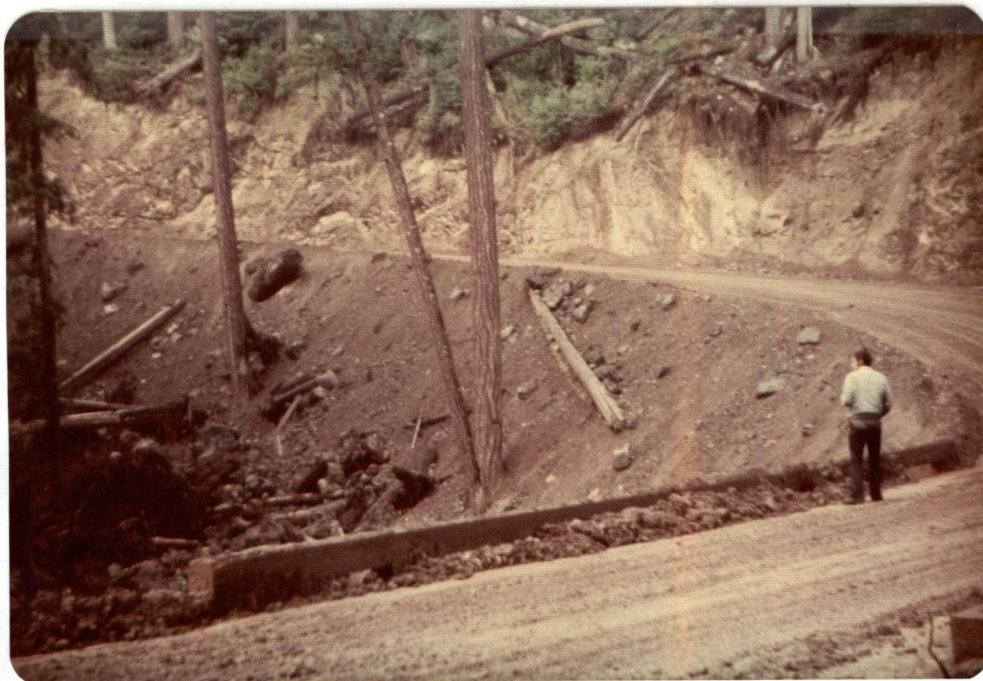
Figure 19. Koksilah sidecast that caused the stream sedimentation seen in Figure 1 (Sept., 1976).
