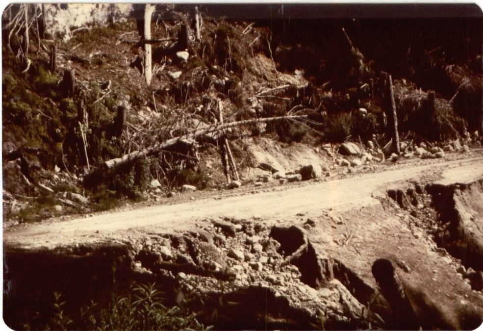
Figure 4. Gully formation cutting into road surface.
