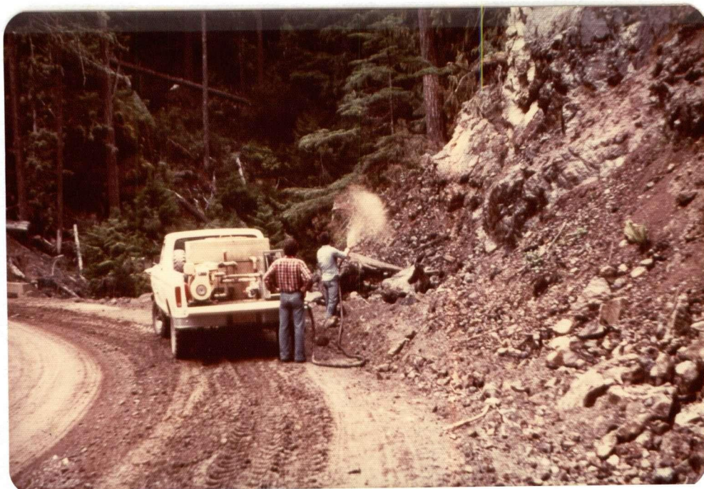
Figure 5. Small (950-liter capacity) hydroseeder used in experiments.
