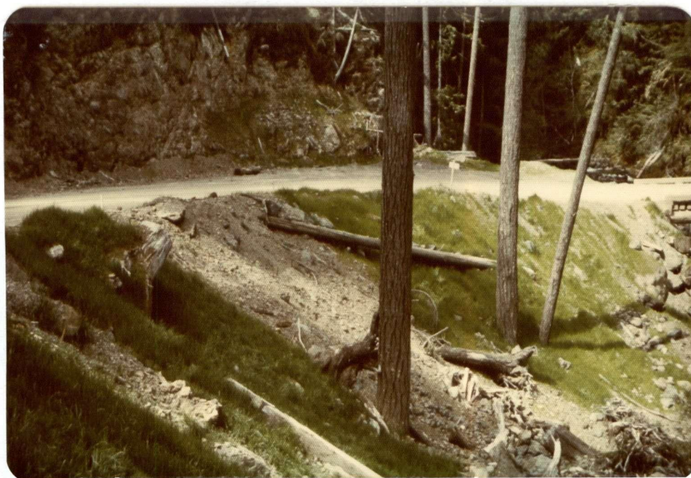
Figure 20. Same sidecast slope in April 1977. Note untreated control area between hydroseeded plots.
