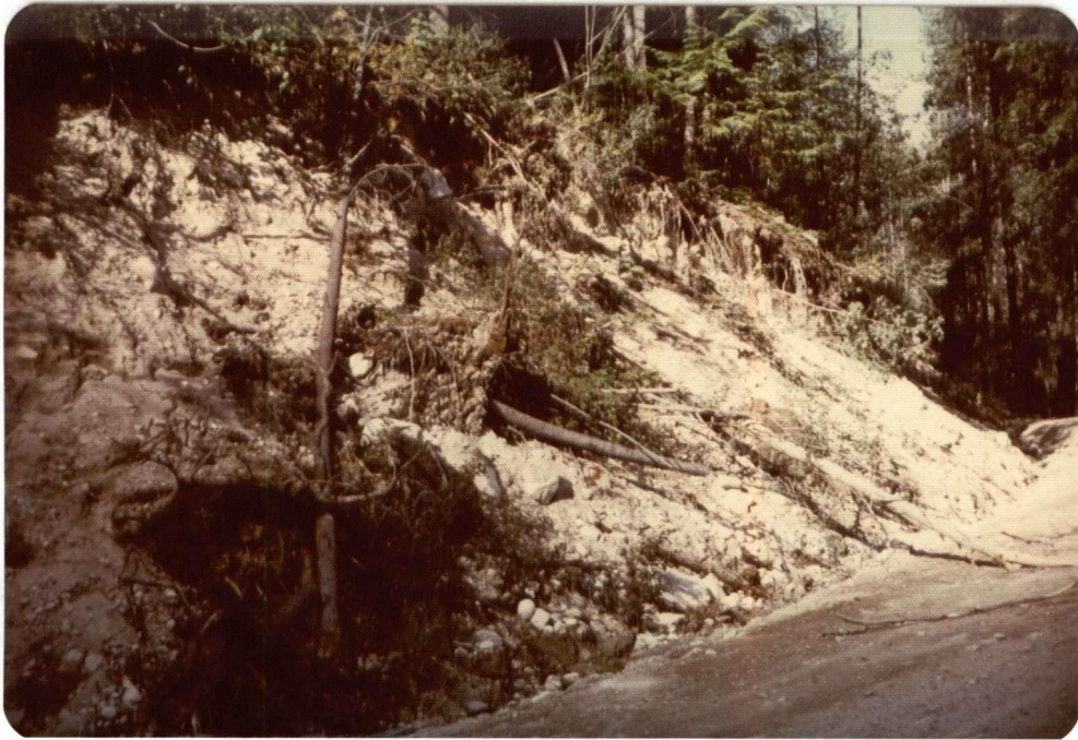
Figure 3. Erosion undercutting forest road bank.
