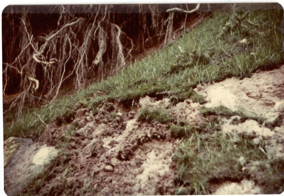
Figure 16. Frost action on Koksilah cut-slope, Jan. 1977.
