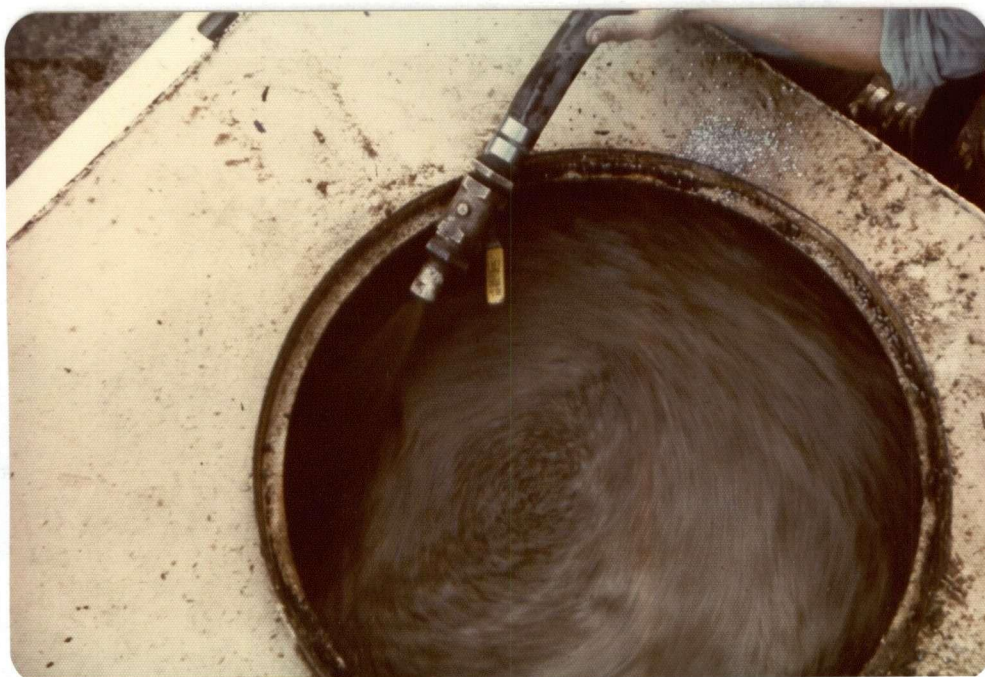
Figure 6. Hydro-slurry containing seed, fertilizer, binder, and mulch.
