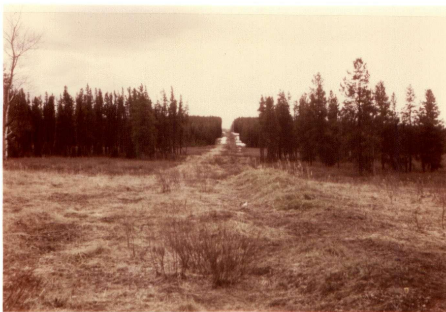
Figure 12. Warmth generated by the underground transportation of natural gas stimulates early spring growth of herbs and grass.
