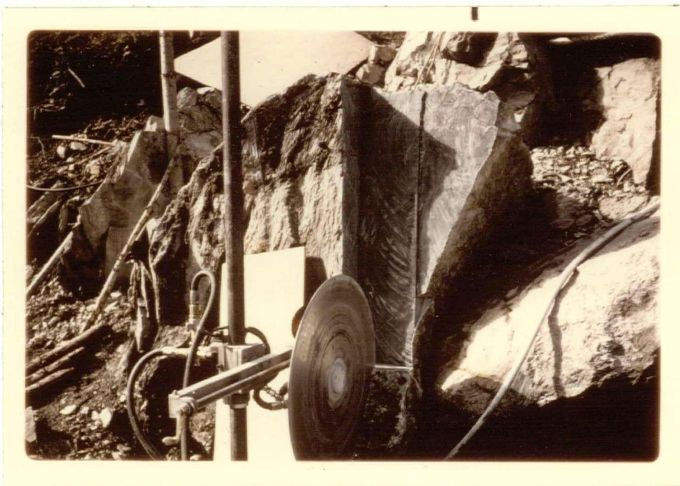
Plate 16: A portion of the nephrite outcrop at O'Ne-ell Creek. In this deposit, the nephrite was removed from the outcrop by means of the specially designed diamond saw shown in the foreground. The saw blade is three feet in diameter.
