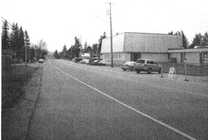
Photo 6.1a Draper Street in front of Hatzic Elementary School (Mission) has one lane of travel in each direction and no sidewalks. A paved shoulder and adjacent gravel parking strip widen the street significantly for the purposes of crossing, and encourage higher speeds. (Photo: Ren Thomas)
