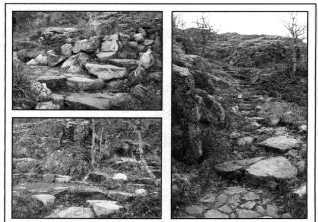
Figure 4.3 Christmas Hill, Victoria. Staircases are built out of stones found on site and take advantage of their natural setting
