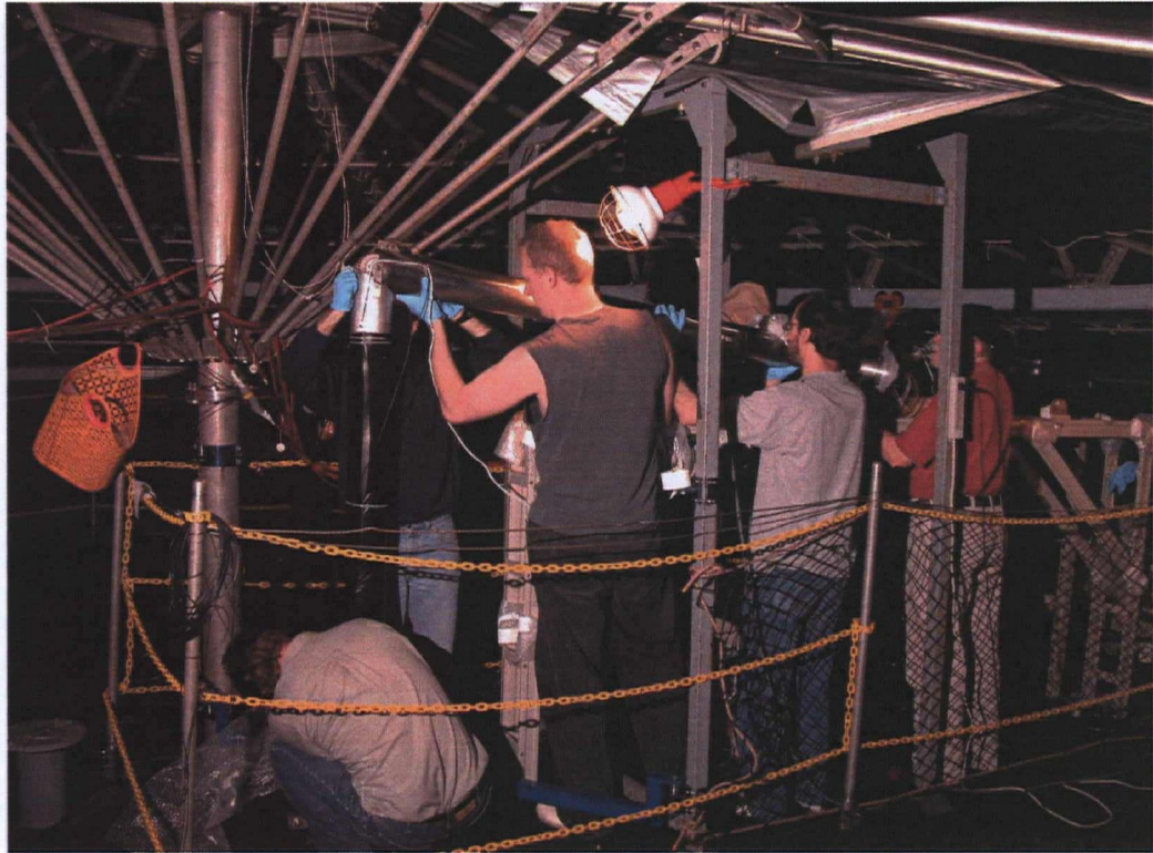
Figure 3.18: Before lowering part 2 of the VS into the 1KT the clamp holding parts one and two straight must be fastened.
