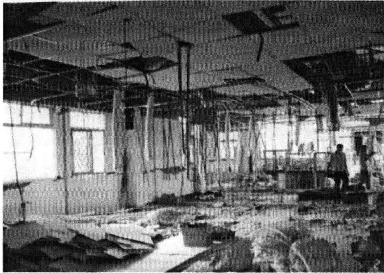
Figure Seven: Nonstructural Damage to PCH Building B
