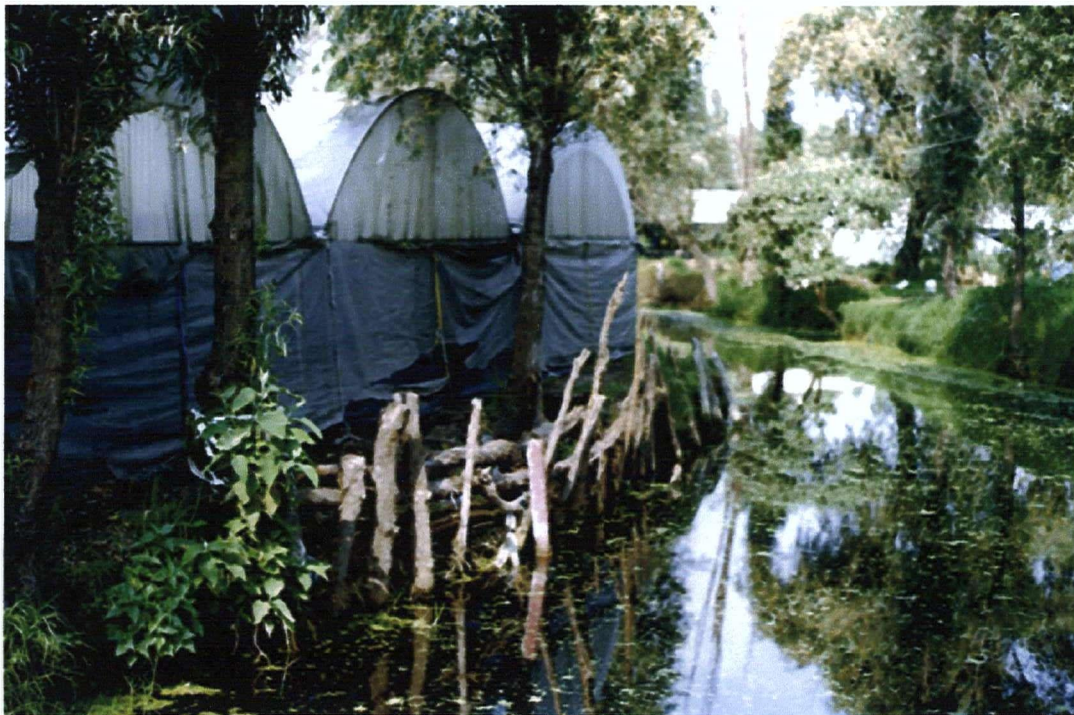
Figure 13. Water running down from the greenhouse roofs has damaged the canal edge, now supported with poles and branches.
