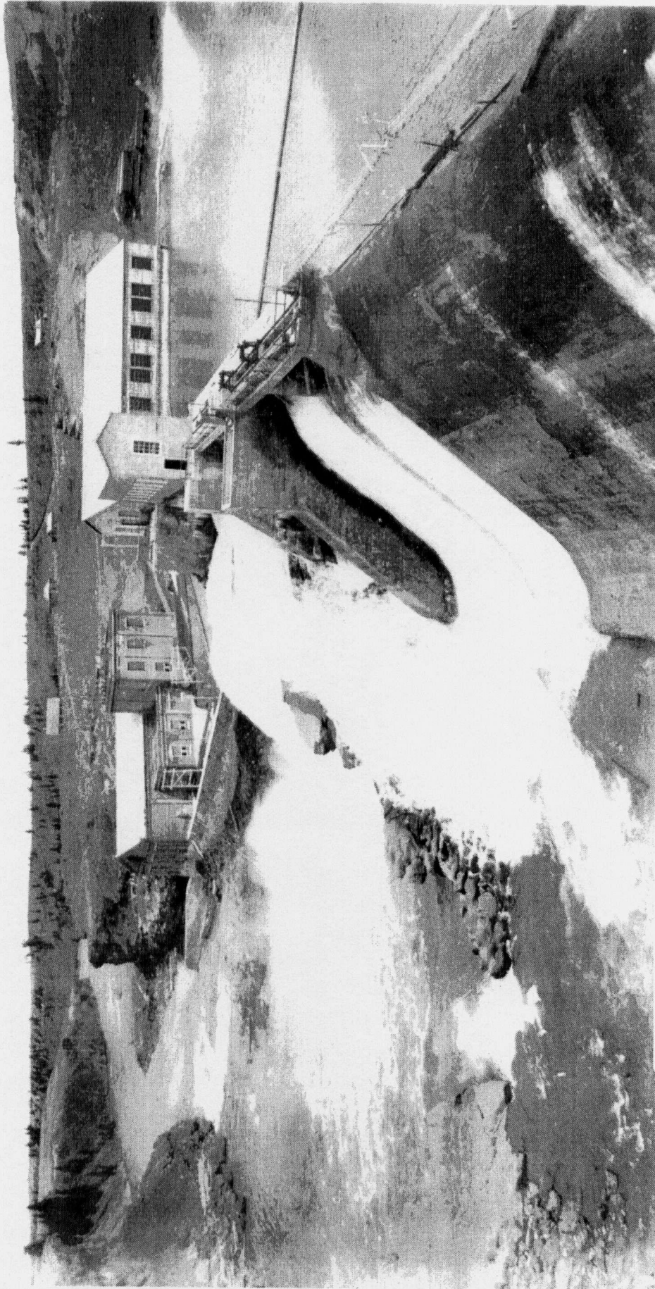
FIGURE 2. Kananaskis Dam (c. 1914) on the Soney Reserve. In 1914, the Calgary Power Company completed this solid concrete dam at the confluence of the Kananaskis and Bow rivers in order to supply power to Calgary.
