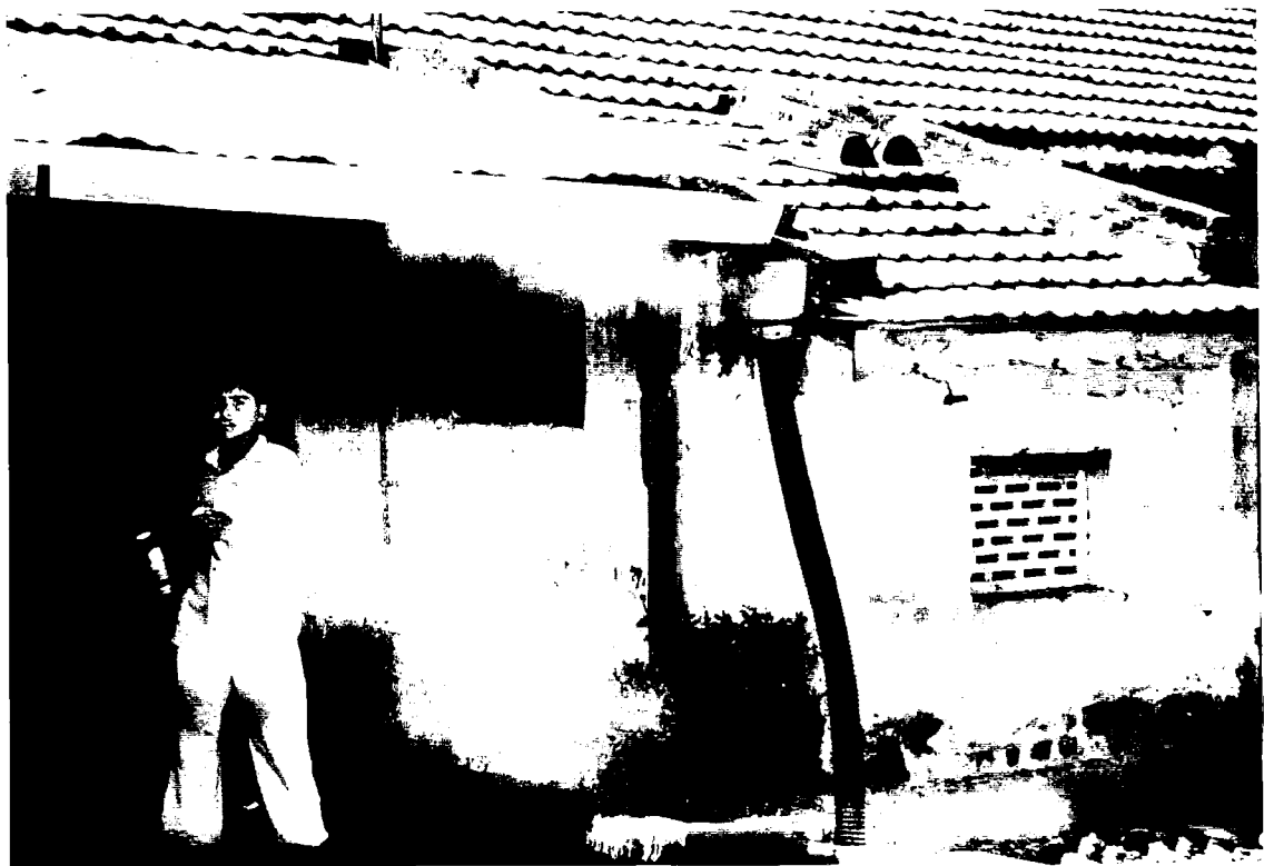
A Roof Water Collection Tank (RWCT) system of a house in a study village in Coastal Bhavnagar, Gujarat. Note the metal shaft running along the roof edge (left) small bucket and plastic piping (centre) leading to underground tank for storage. (Courtesy of John Wood.)
