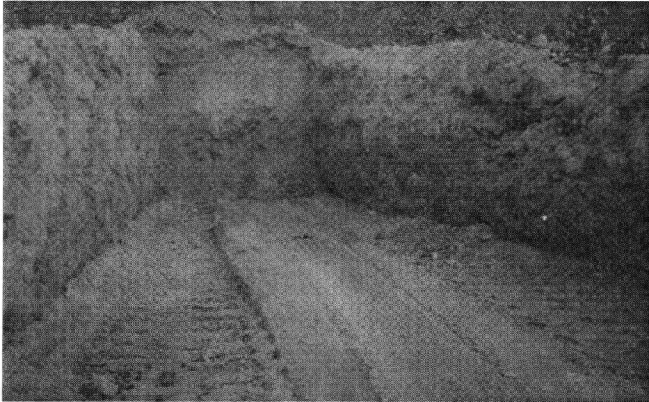
Photograph 21.1: Test Pit Excavation.
