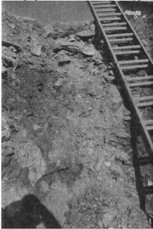
Photograph 16.1: Test Pit Excavation.
