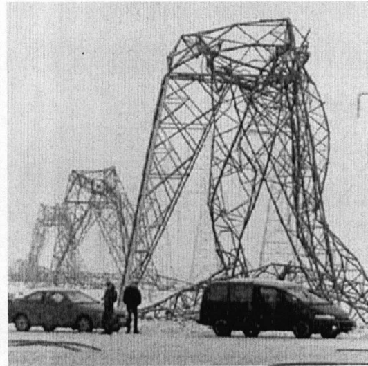
Figure 1.4: Transmission tower failure due to Ice storm, Quebec, 1998.
