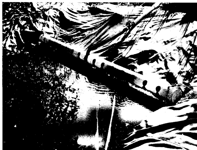
Figure 4-2 Influent inlet, the replaced multi-port inlet, and the influent control valve
