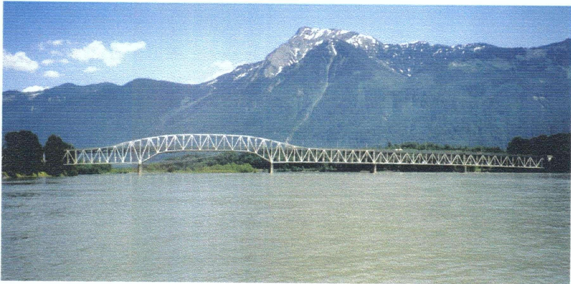
Figure C.1: Fraser River at Agassiz-Rosedale Bridge, facing upstream. Former WSC gauge site 08MF035. Width is 510 m. Described as a wandering gravel-bed river ( D_{50, surf} = 42 mm), with a slope of 4.8 \times 10^{-4} (McLean et al. 1999). If bridge spans are numbered from left to right (facing upstream), the thalweg flows through span 5, and a shallow bar occurs at span 2. All 2000 freshet bedload sampling stations were downstream of the bridge at spans 3 and 4 (Chapters 1, 3, and 4).
