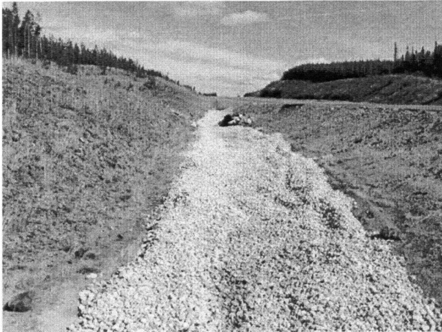
E-6. The newly replaced crushed limestone
