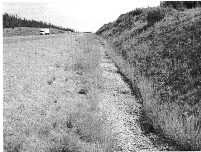
E-3 The south ditch was covered with limestone
