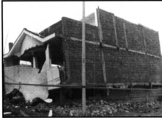
Figure 2-6: Collapse of CM building due to inadequate wall density, 2001 Atico earthquake, Peru (San Bartolome et al, 2004)
