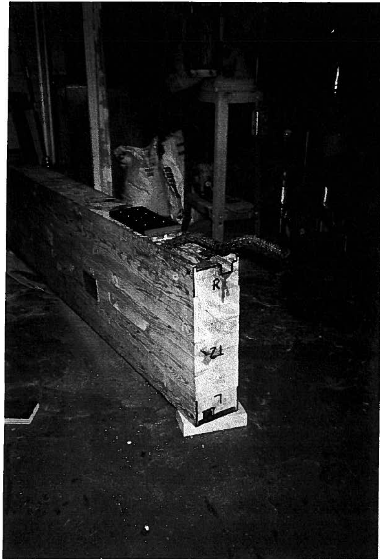
Fig.4.25 Fitting inclined rebars and plates.
