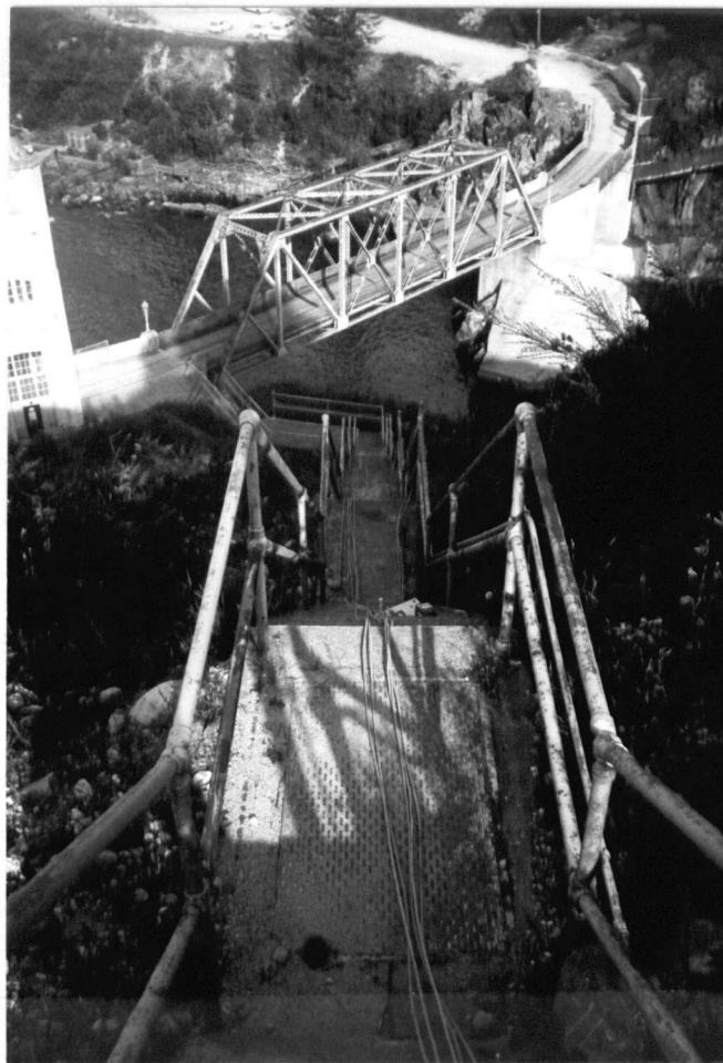
PHOTOGRAPH 9 Looking down stairway on east abutment. Sensors at Node 37 are visible in the foreground. The powerhouse is visible in the left background. RUSKIN DAM AMBIENT VIBRATION FIELD TEST, LOW RESERVOIR, 30 APRIL 94
