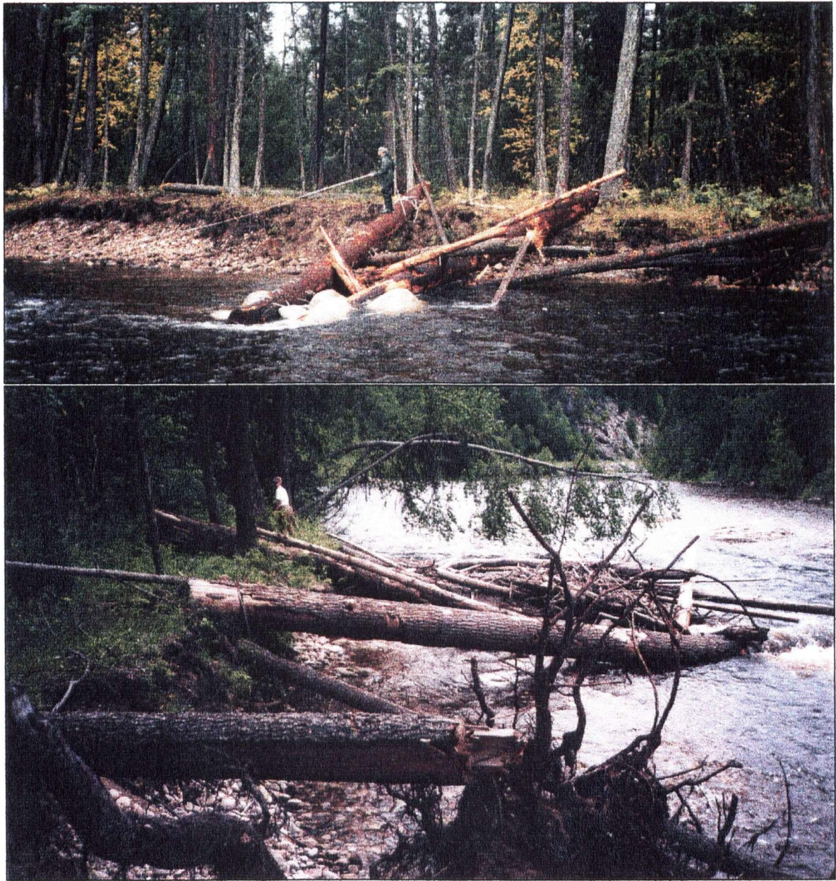
Figure 6-8: WK-8 as built Oct. 1997 (top) and post freshet looking upstream June 1998 (bottom). Note (bottom photo) debris on upstream face, fallen bank anchor tree (centre left) and eroded bank downstream.
