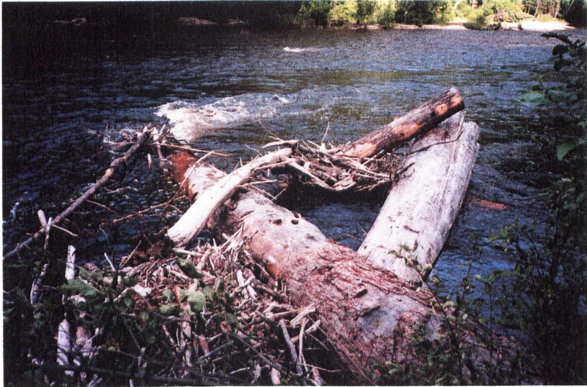
Figure 6-11: Structure WK-9 (looking downstream from bank, flow is left to right). Both LWD pieces oriented roughly parallel to flow (centre right) increase the structure debris capture efficiency.
