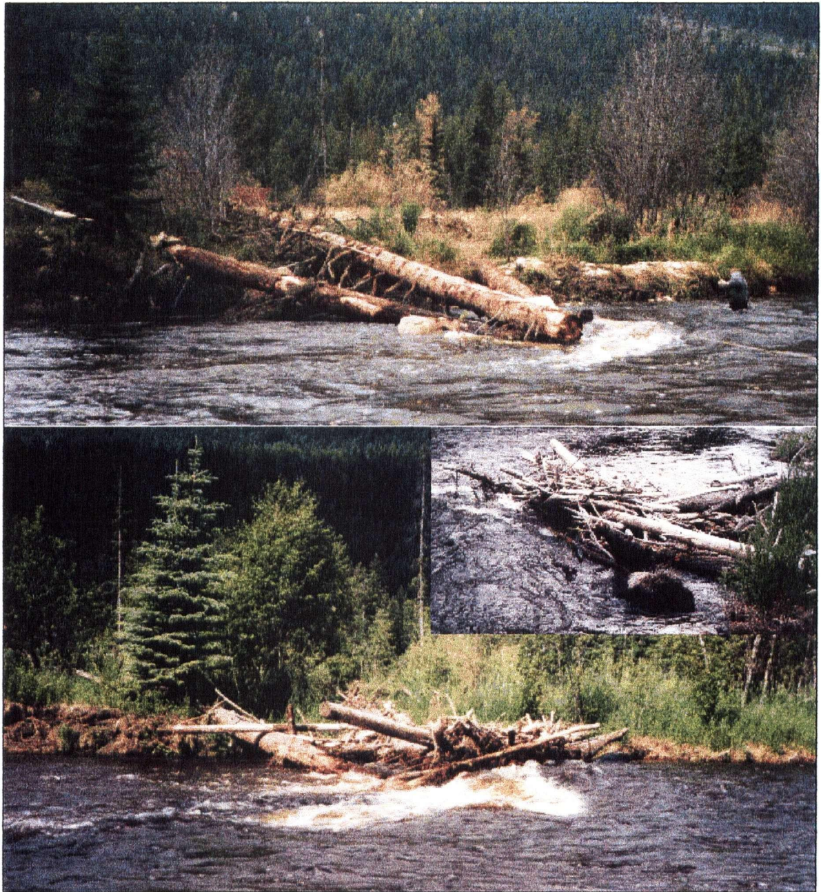
Figure 6-7: Debris accumulation on face of WK-1 structure. As built - Oct. 1997 (top, note human figure at right for scale), post freshet - June 1998 (bottom) and looking downstream from bank (inset).
