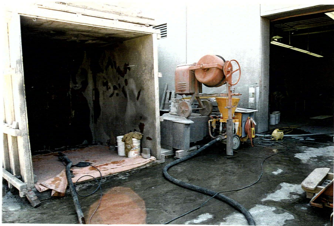
Figure 5.9 Dry-mix shotcreting.
