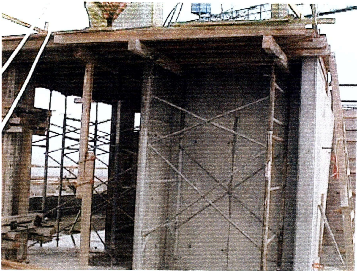
Figure 3.10 Typical Formwork
