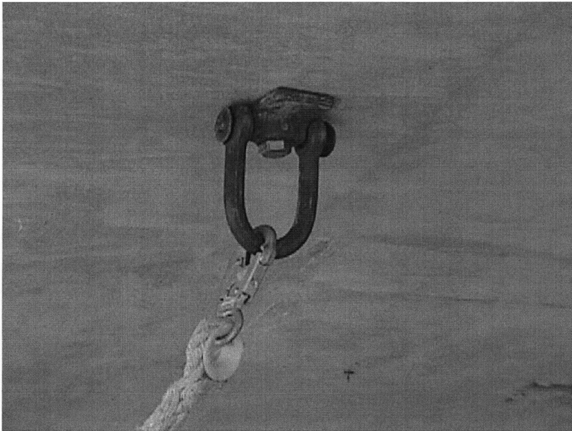
Figure 3.16 Tie-Off Anchor in Ceiling
