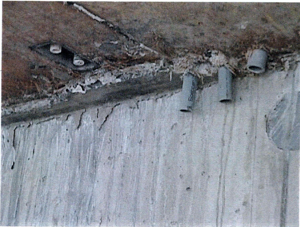
Figure 3.4 Rough Ceiling Finish
