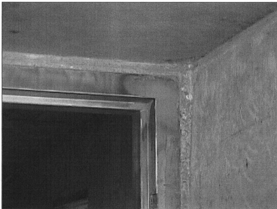
Figure 3.7 Misaligned Door Frame
