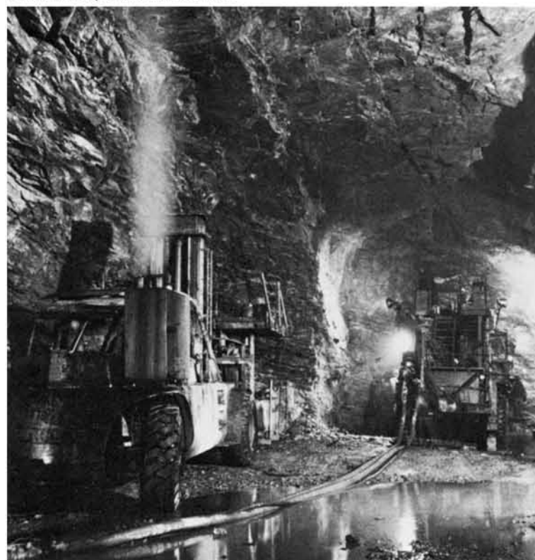
Excavation of the diversion tunnel prior to construction of the Revelstoke dam.
