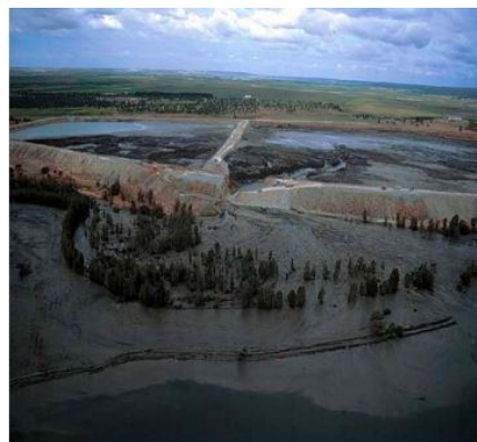
Figure 5. Los Frailes tailings failure (Ref http://en.wikipedia.org/wiki/Dam_failure )
