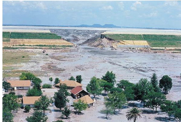
Figure 3. Merriespruit tailings failure (www.infomine.com)
