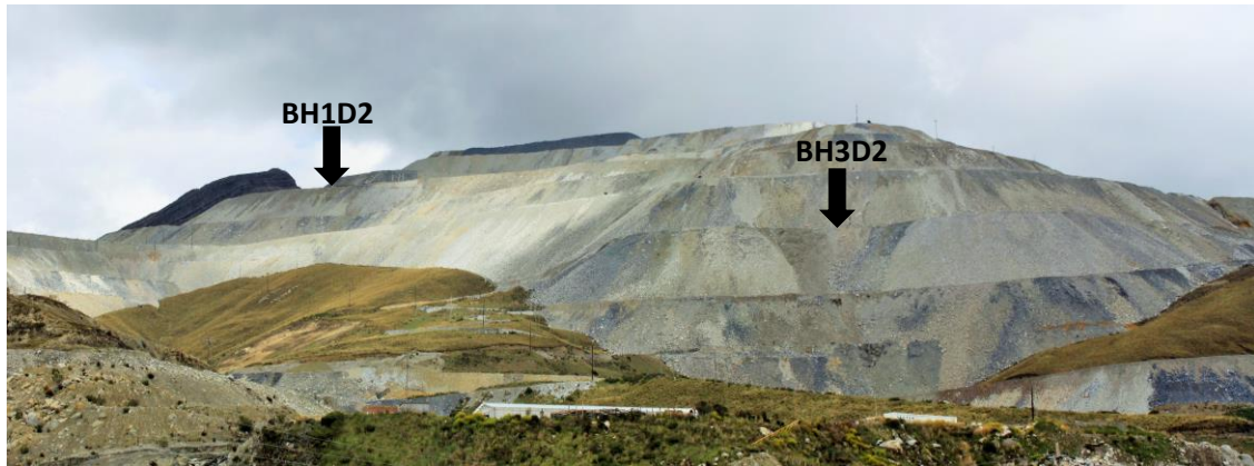
Figure 1 Borehole location on the East Dump at Antamina.
