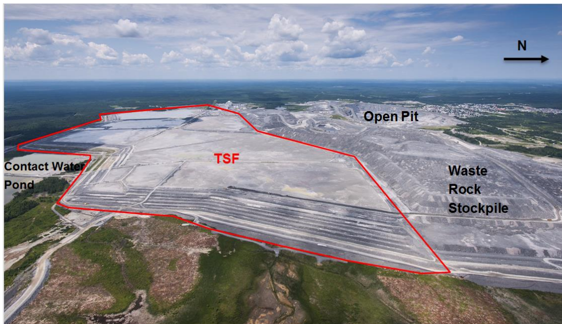
Figure 1. View of the Canadian Malartic Mine in 2015, looking west.
