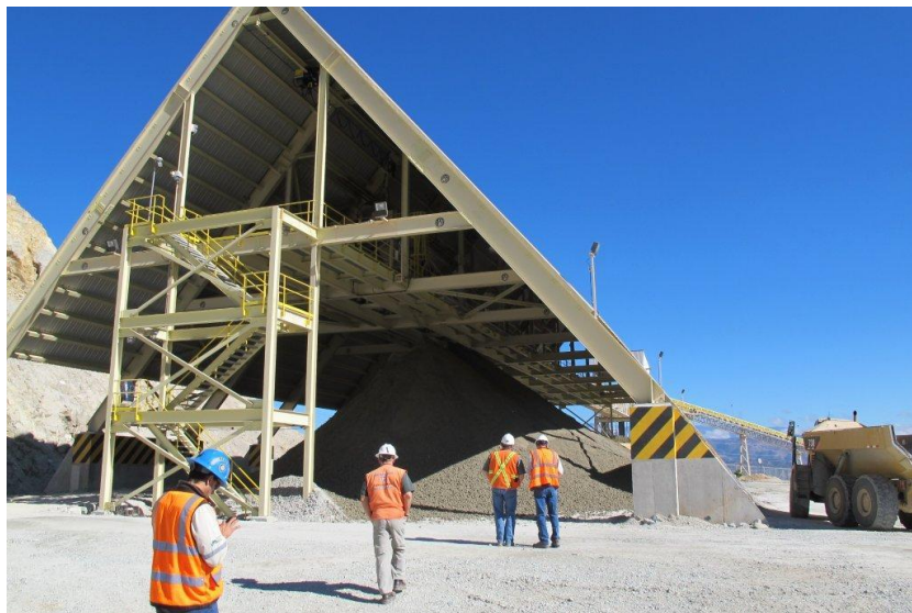
Figure 2. The roof over the stacker pad of the Marlin Mine, Guatemala filter press tailings facility.
