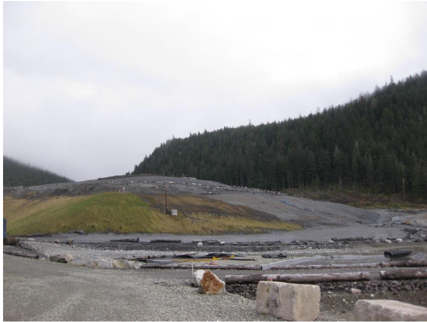
Figure 9. The Greens Creek filter press tailings stack showing the outer slope on which vegetation has established naturally.
