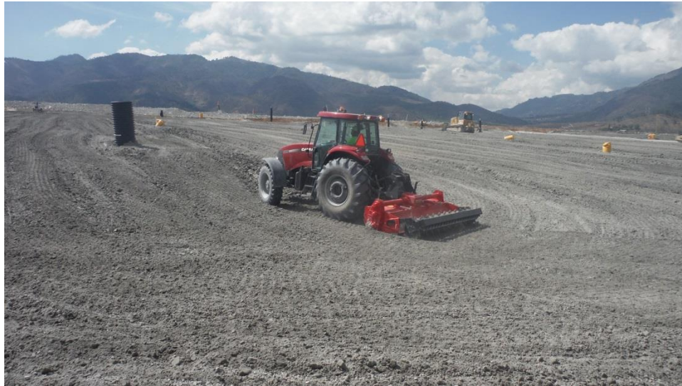
Figure 3. Filter pressed tailings in place and being disked to reduce moisture content.
