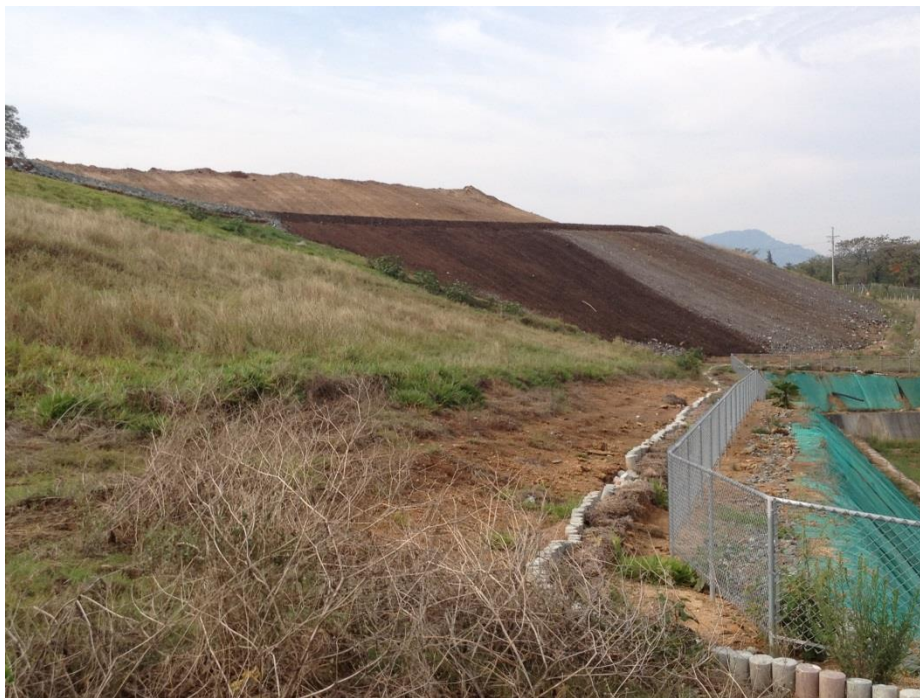
Figure 6. The outer face of the Escobal Tailings Stack. Here the tailings rise above the waste rock that is partially covered with soil and to the left already supporting vegetation.
