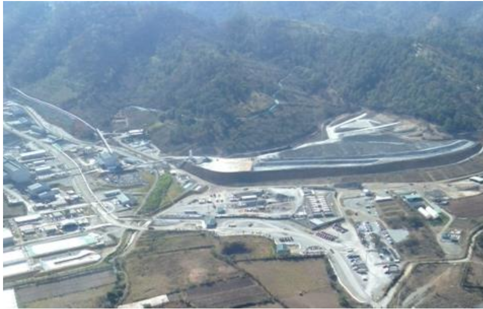
Figure 5. The Escobal Tailings Stack. In the foreground is the perimeter embankment made of waste rock that is covered soon after placement with topsoil and vegetated.
