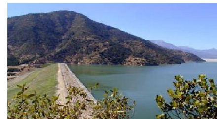
Caren Tailings Impoundment - Rancagua - El Teniente Mine
