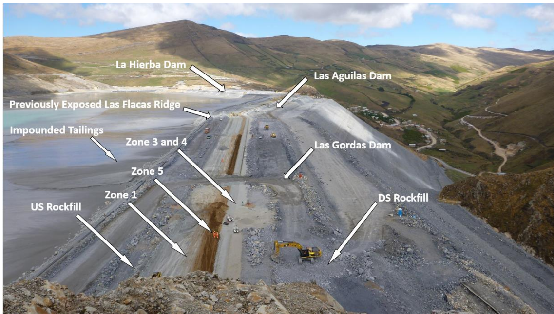
Figure 1. TSF Dam with Noted Zonation (Approximate elevation 3765 m)
