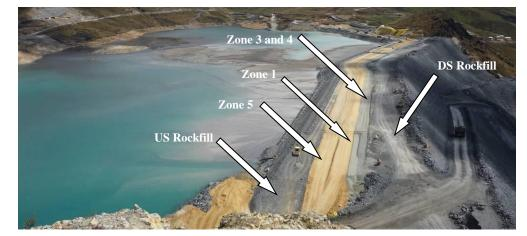
Figure 7: TSF Dam Crest During Stage 5 Construction
