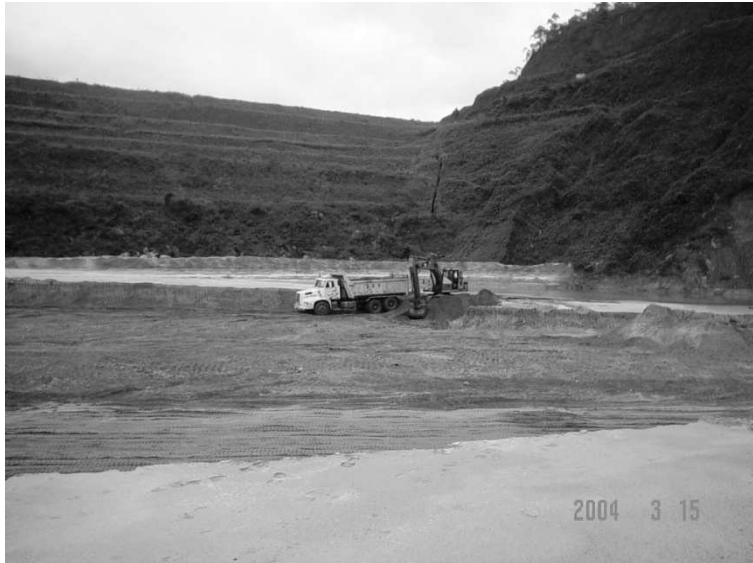
Photo 1- View of the tailings surface after a few days of stopping the discharge.
