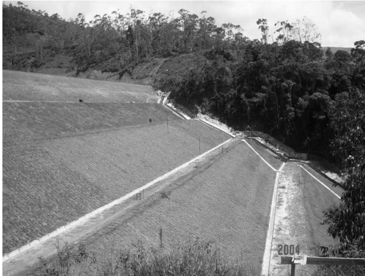
Photo 3- View of the final slope surface of the Germano buttress that is progressively prepared for closure.
