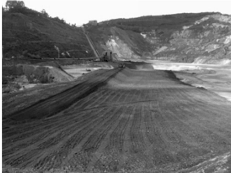
Photo 6- View of the Germano Pit drainage blanket in construction.
