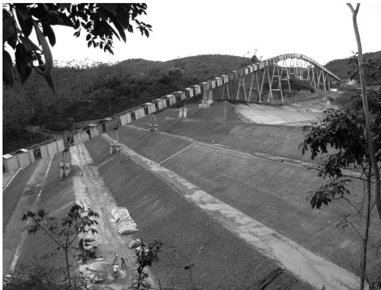
Photo 4- View of a conveyor belt structure resting upon the final slope surface of stacked tailings.
