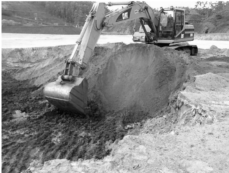
Photo 2- View of the tailings surface being excavated to obtain material to raise the structure.
