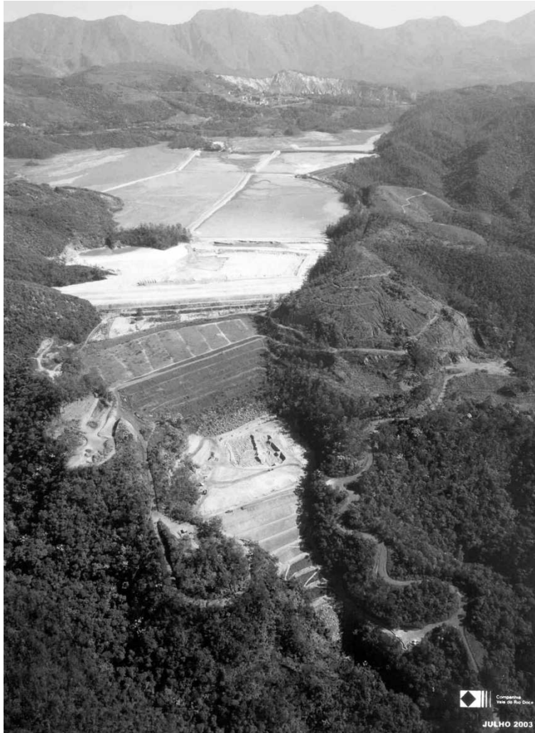
Photo 5- View of the Germano buttress at an early stage of construction.
