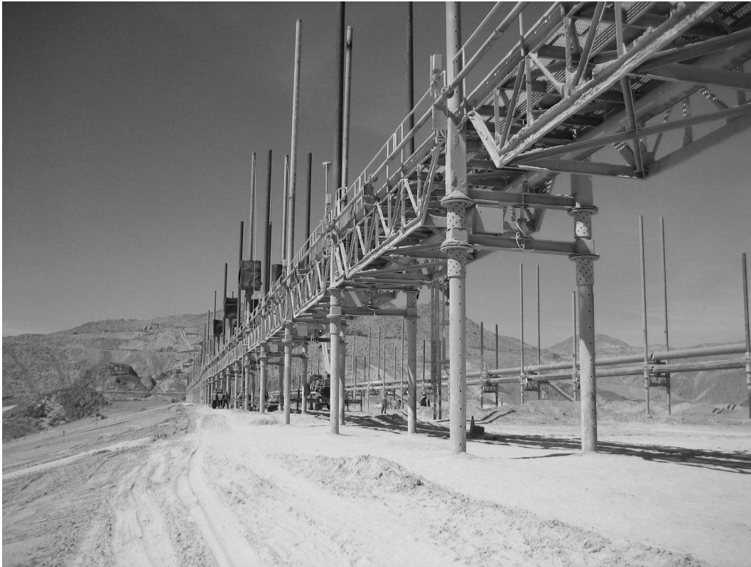
Photo 1: Jacking Header
