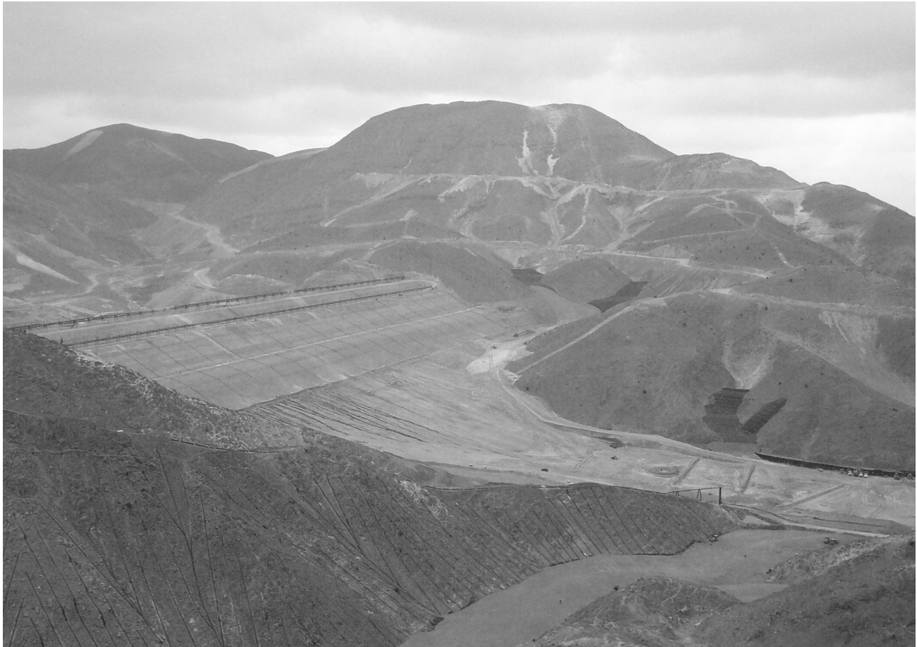
Photo 3: Starter Dam and Initial Underflow Deposition
